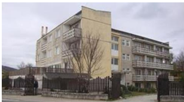
Fig.2 Dormitory in M.Tarnovo – S/E view
